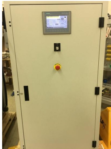
Fig.5. Front door of the APT-100-3 DC module with advanced control system
